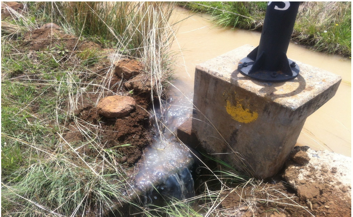
Photo 5.5: Overflow of the A canal due to siphon blockage
