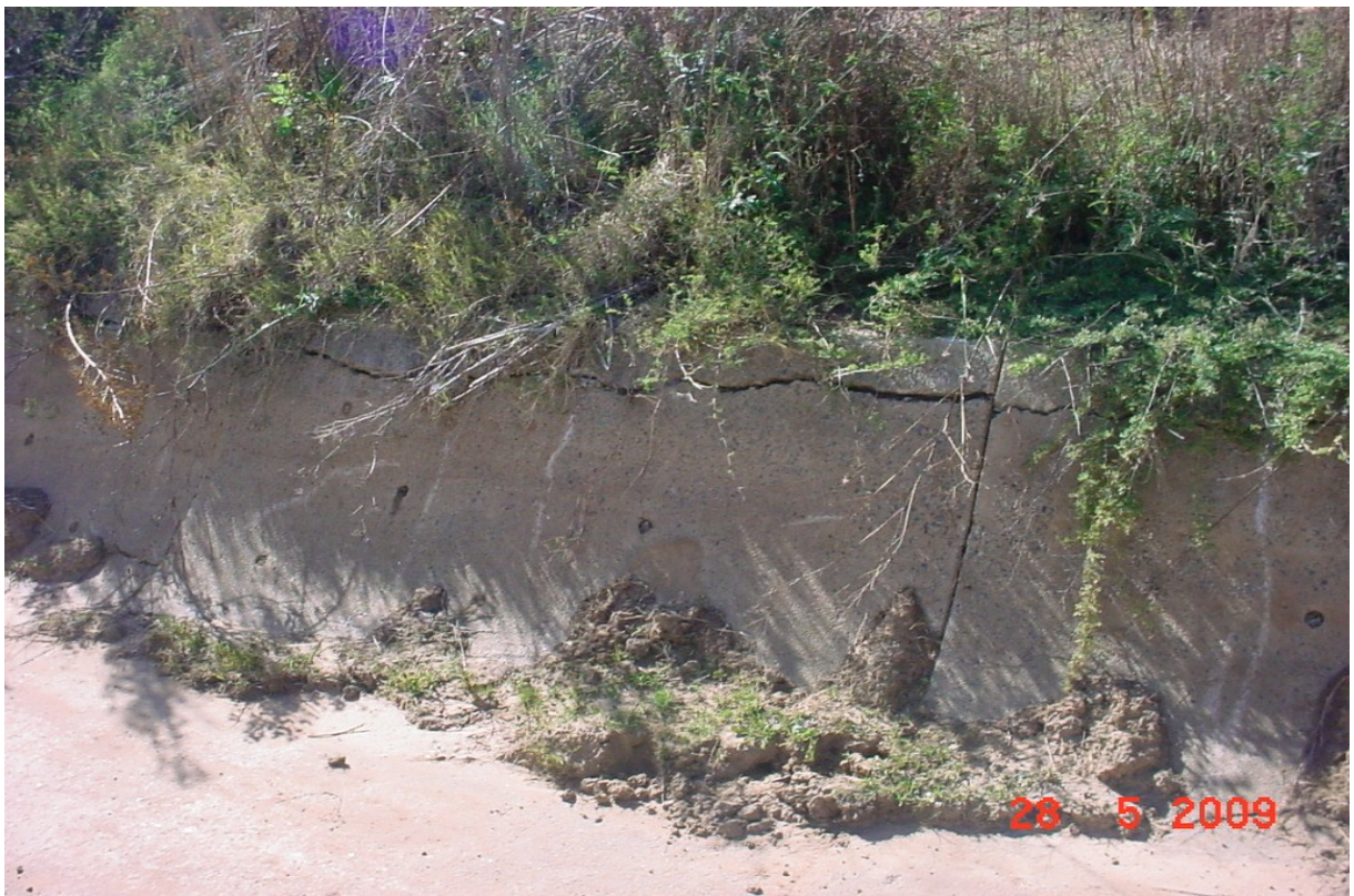
Photo 5.2: Major Cracks on the S canal as well as vegetation growth in the joints of the concrete panels
