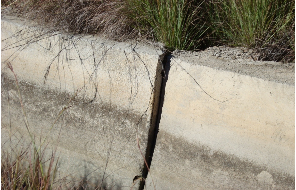
Photo 5.1: Open joints between the concrete panels as well as growth in the canal
