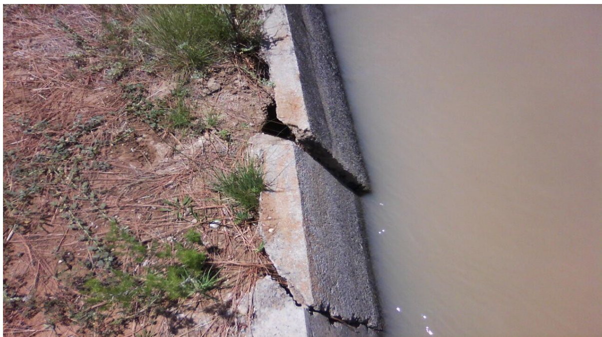
Photo 8.1: Broken section of concrete panels of canal system
