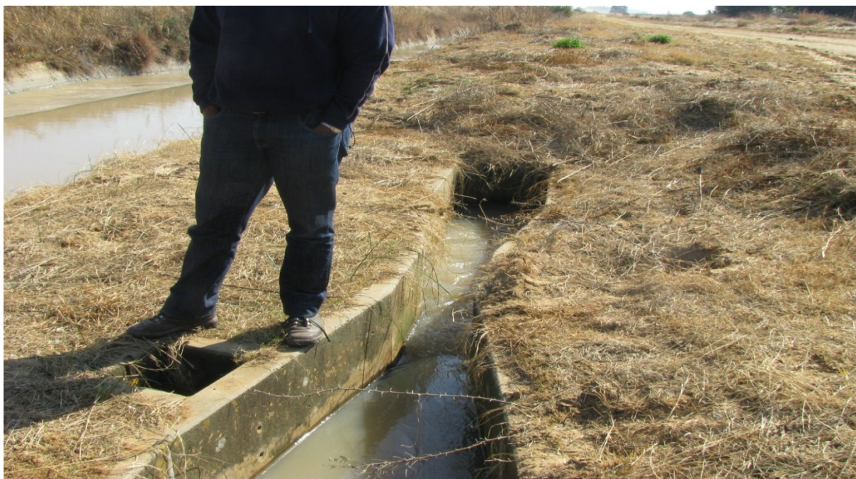
Photo 8.3: Potential for submergence increases inaccuracy in Parshall flumes
