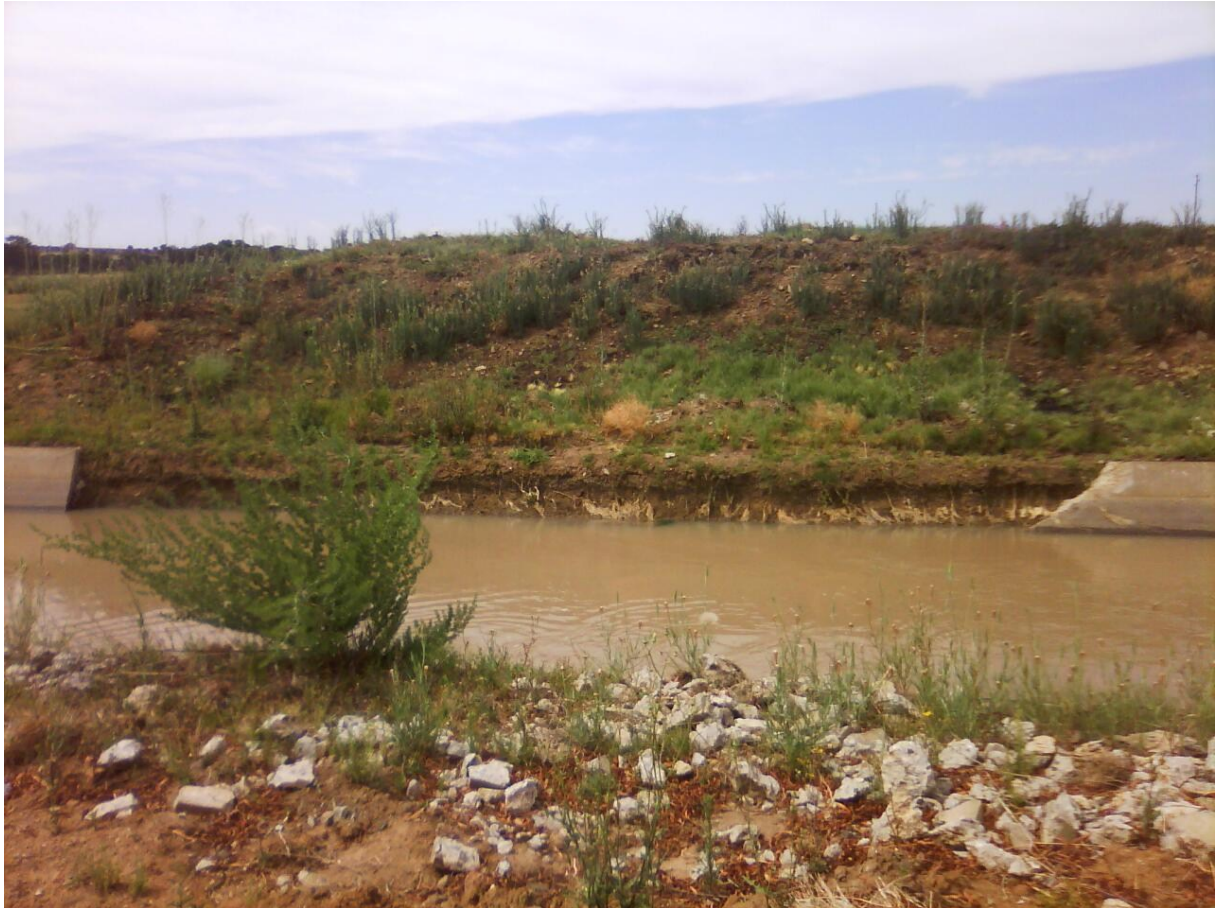
Photo 5.7: Concrete panels in the V canal eroded due to drainage problems
