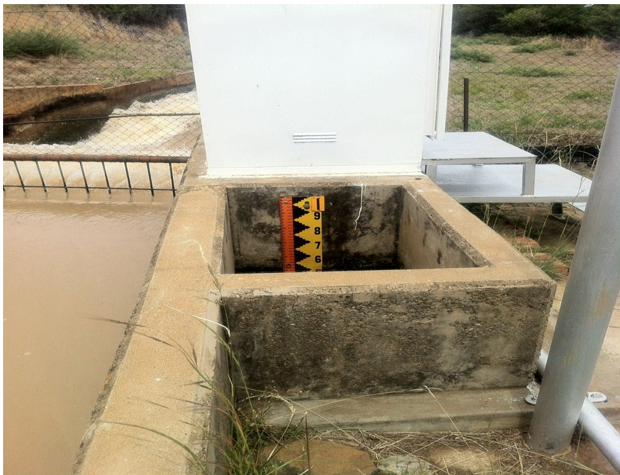
Photo 4.3: Photo of the flow gauging station into Sand River main canal downstream of Allemanskraal Dam
