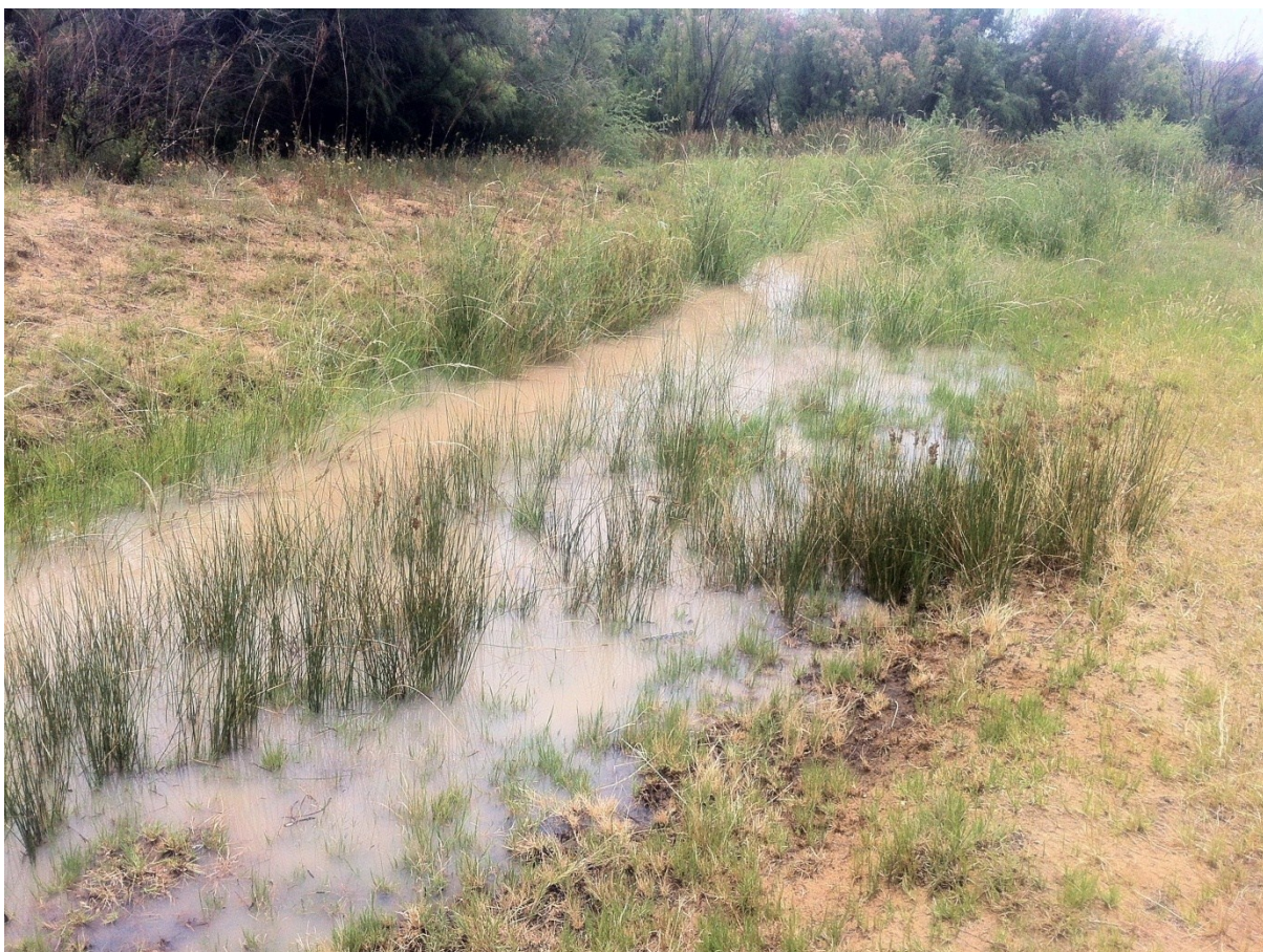
Photo 5.6: B canal spilling as a result of siphon blockage
