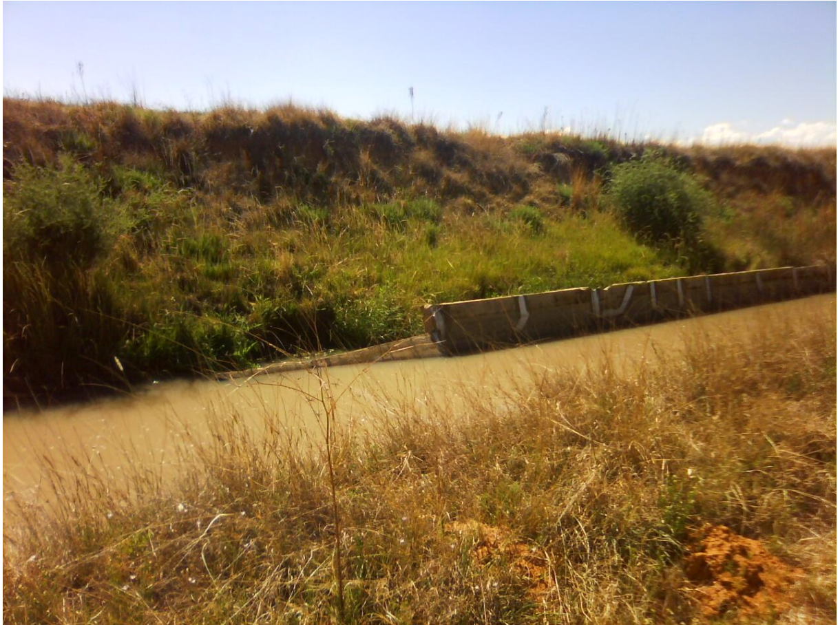
Photo 5.8: Concrete panels missing on the V canal including extent of repairs
